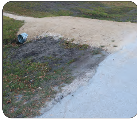
Older adults who need walkers or canes or who have low vision have difficulties navigating sections of uneven pavement that slopes off into a ditch and has gravel and ruts.
