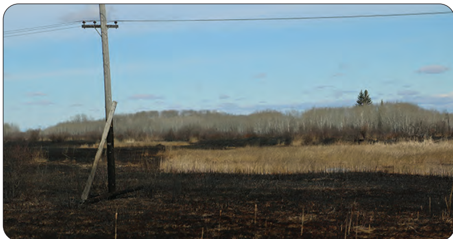
Highway 68 west of Poplarfield is shown after a wildfire swept through in April 2018, burning Hydro poles, grasses and trees.
