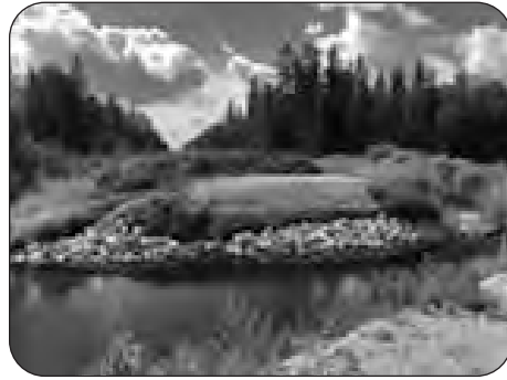
The province placed rock along the bank of the washout.
