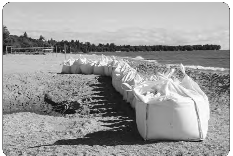
The RM of Gimli placed super sandbags at a town drain on Gimli Beach to prevent waves from swamping it.
