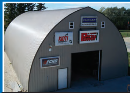
Quality Domtek Roofing installed over old metal
