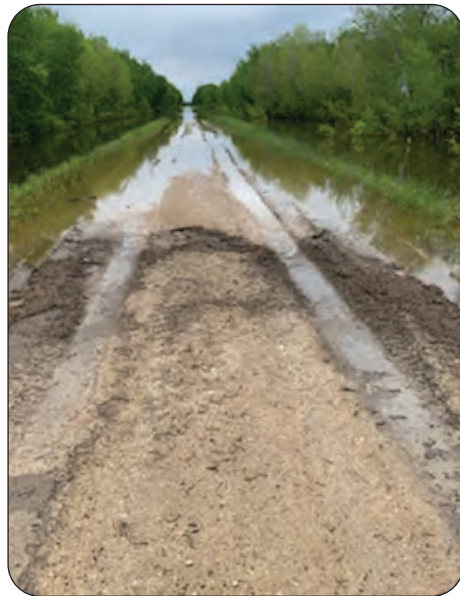
Bifrost-Riverton council authorized road repairs, but the water hasn’t receded.
