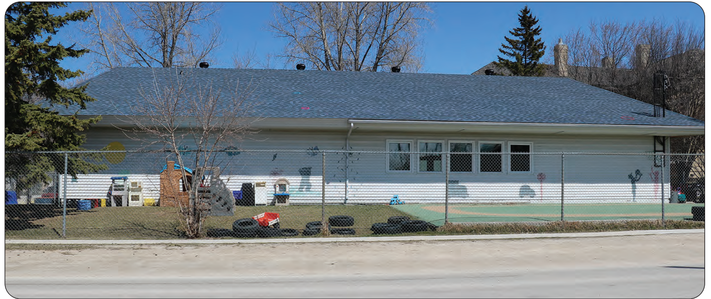
Gimli Children's is in the process of undergoing renovations.
