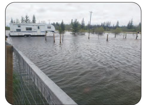
The water backed up west of PR 222 at Spruce Bay Road.
